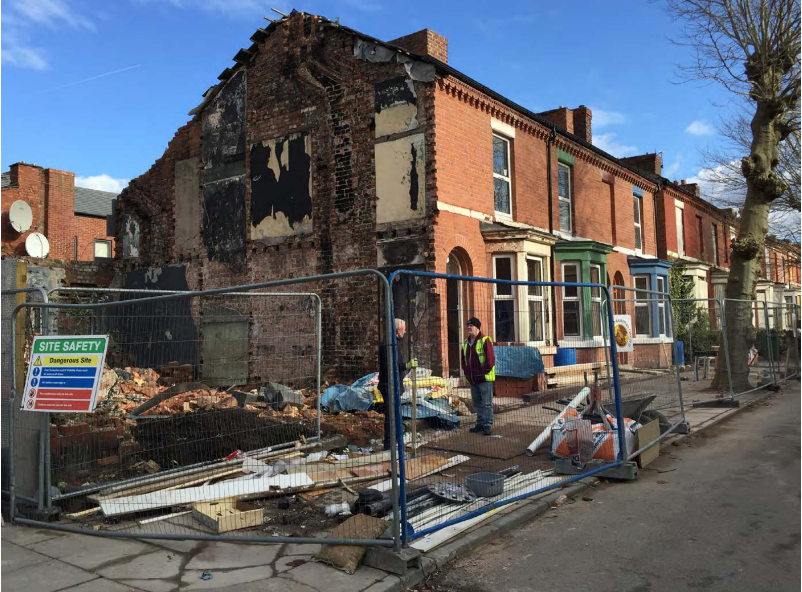
Construction works. Photo © Eutopian
